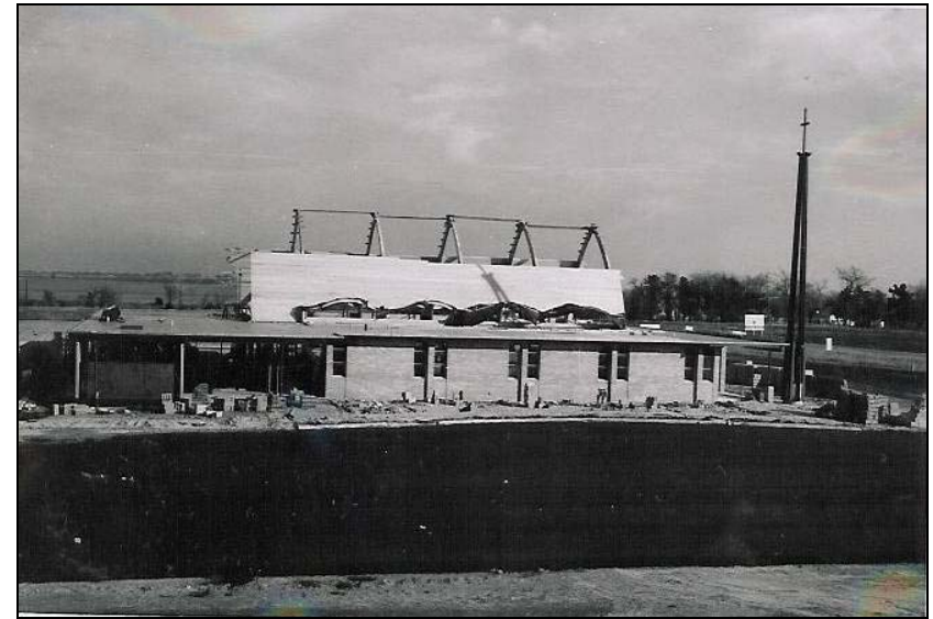
Building progress on Campbell Road
