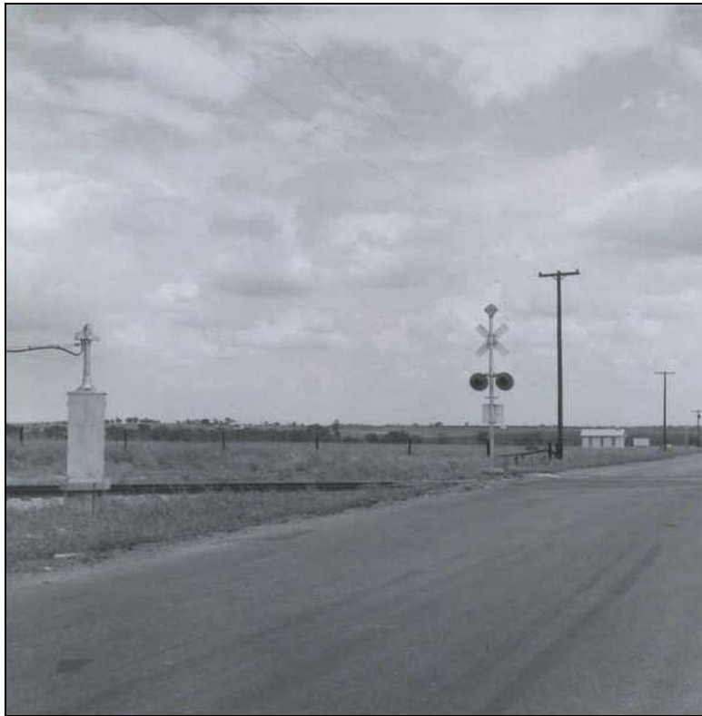
Looking east, west of the rail road tracks on Campbell Road
