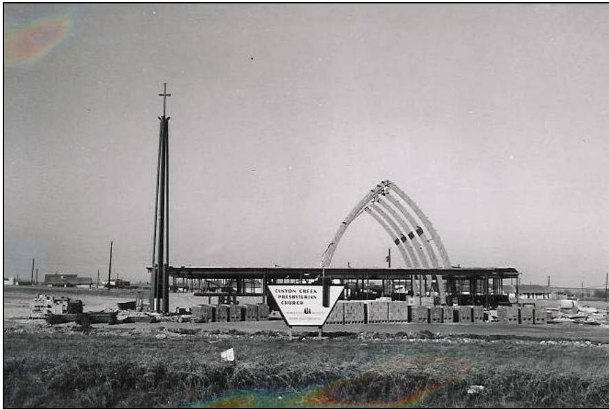
Building progress on Campbell Road.
