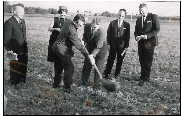
Groundbreaking on Campbell Road
