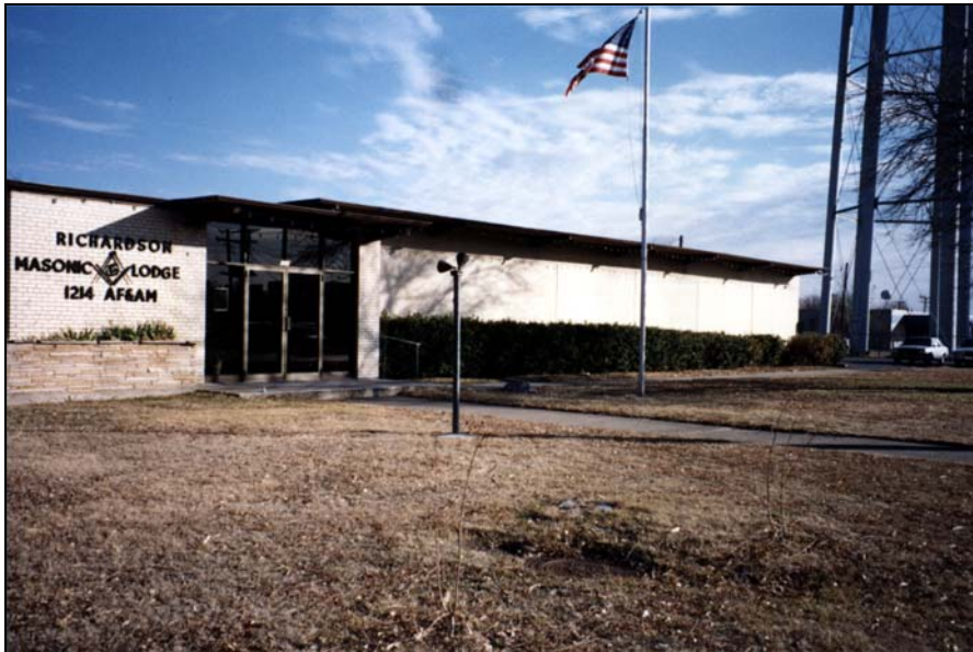
Site of the first worship service, November 25, 1962
